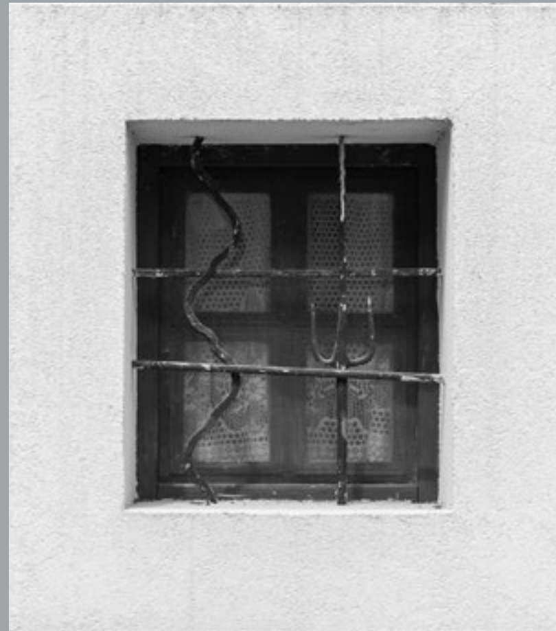
Window grill, 28 Bartók Béla Street, photo: 2022
